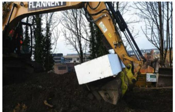
investigation found the lifting operation had not been properly planned and the block was simply held between the arm of the excavator and the bucket.
